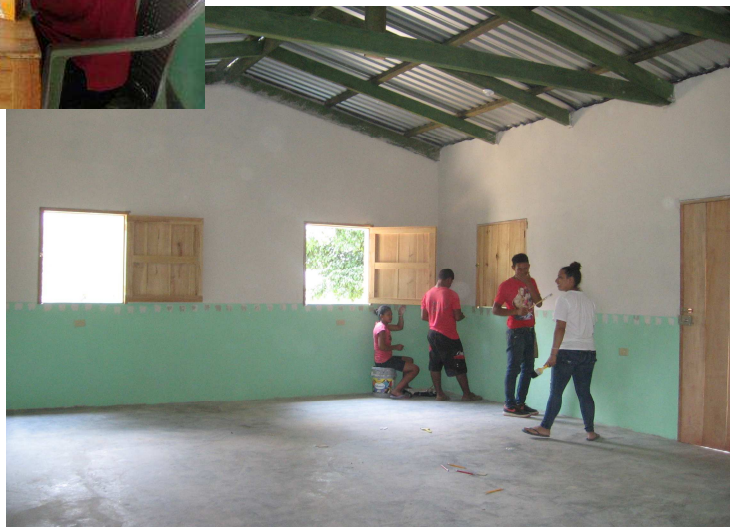
Fuerza students painting the interior of the newly constructed dental clinic
