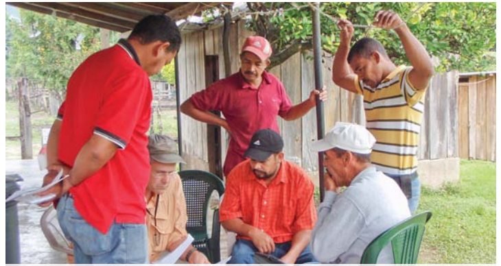
Nelson and Brad plan construction of the Dental Clinic
