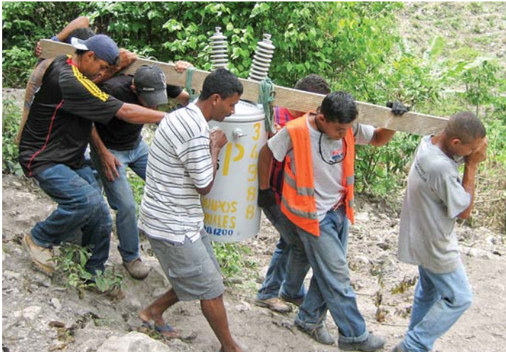
The men struggle with key equipment for the new water system
